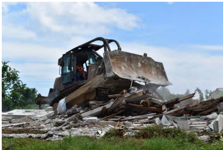
An 850J dozer clearing an old accommodation block at Lombrum Naval Base.
