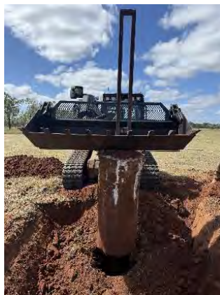
Pozi-track SSL installing a Windsock at Macrossan Airfield, Townsville as part of Ex Global Dexterity 25.
