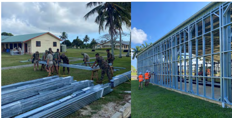
The Exercise Povai Sapper 25 contingent work alongside HMAF engineers building steel frames as part of the gymnasium upgrades.
