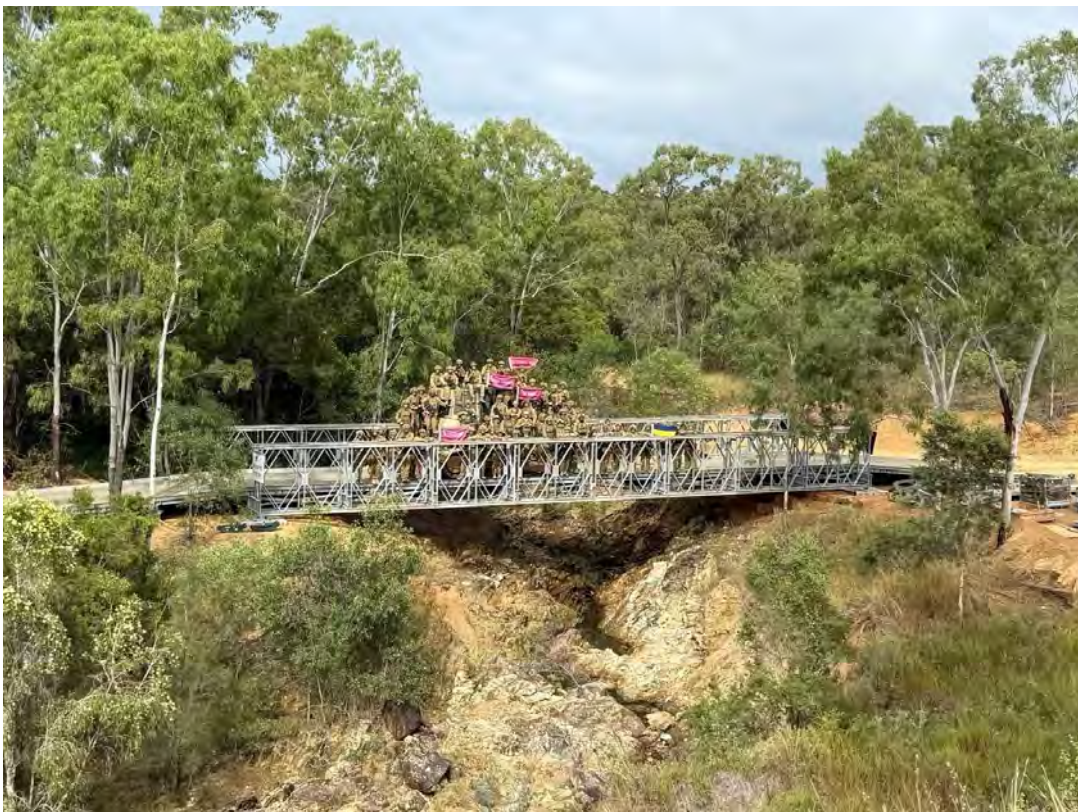
17 Construction Squadron's Fixed Modular Bridge
