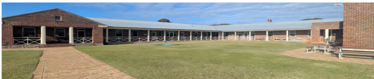
Kingston Barracks, Rottneest Island post refurbishment by members of 13 ER
