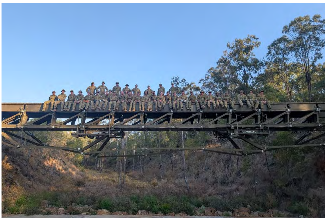
11 CES Members upon completion of MGB construction
