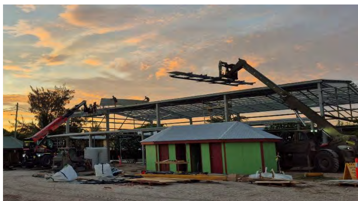
2 TP construction of the portal frame on Poruma Island.
