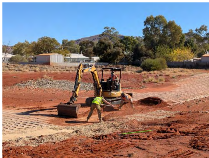
Image 2 – CPL Volta, SPR Bell and SPR Carbone battle the flies whilst conducting defects rectification works on the Flood Management System in Amata.
